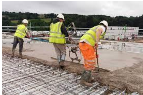
Figs (xxv) (xxvi) pouring in situ concrete on permanent metal deck formwork
