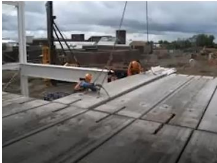
Figure 7 – Precast concrete floor
