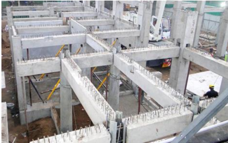
Figure 2 – In-situ concrete frame
