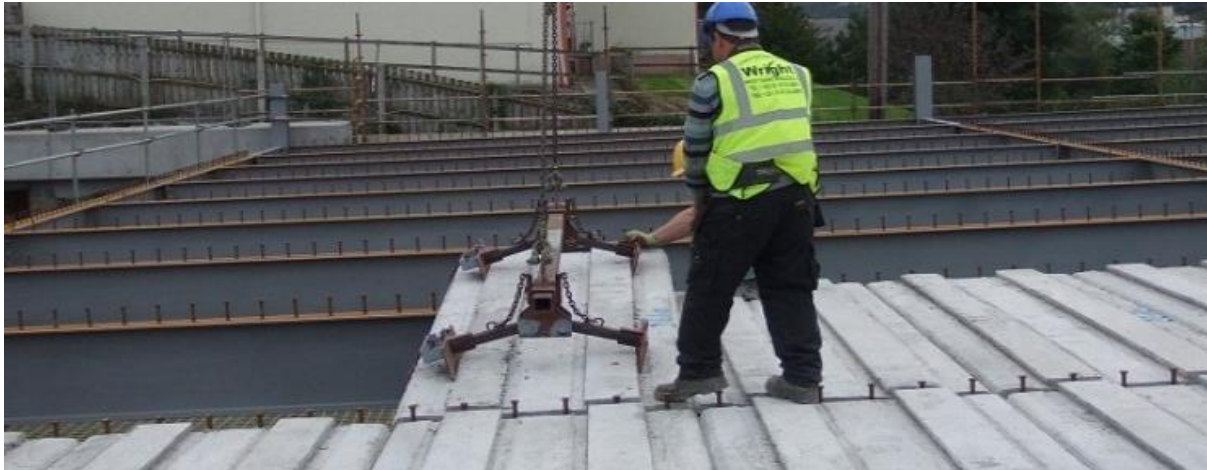
Figure 8 – Composite plate flooring
