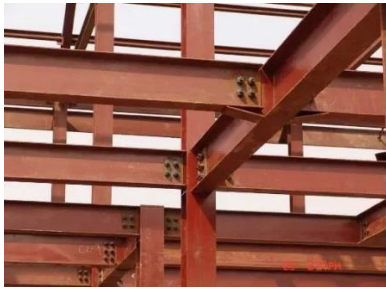
Fig (i) Steel Connections
