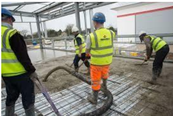
Figs (xxv) (xxvi) pouring in situ concrete on permanent metal deck formwork
