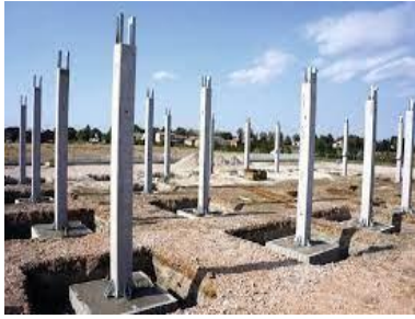
Fig (vii) PCC Columns on bases
